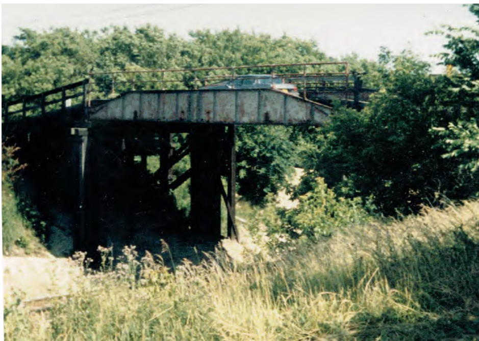
East Norwich Avenue Bridge
