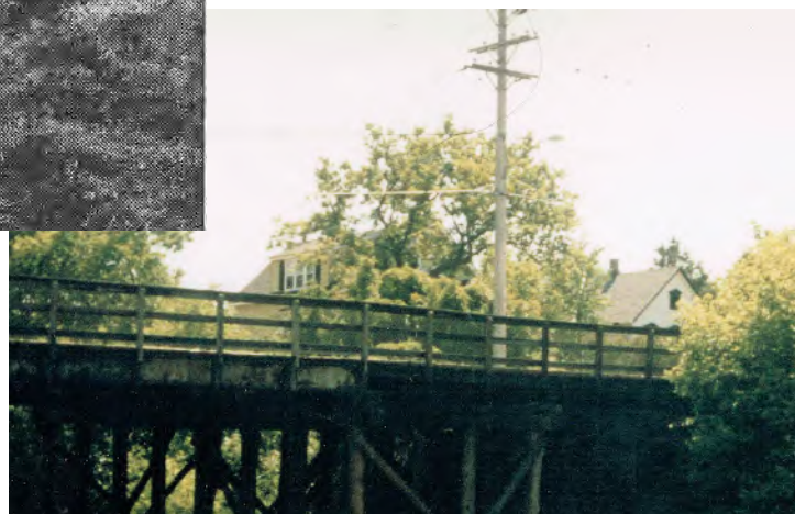
East Tripoli Avenue Bridge
