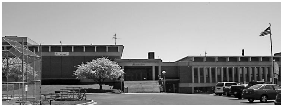
St. Thomas More High School addition at 2601 E. Morgan Avenue.
