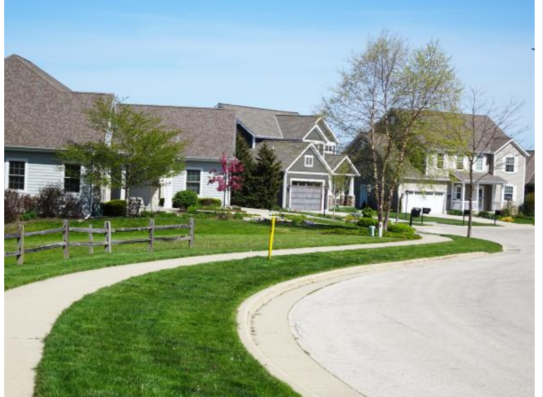
These homes in Trestle Creek Subdivision, built about a decade or so ago, replaced Karen's baseball field.
