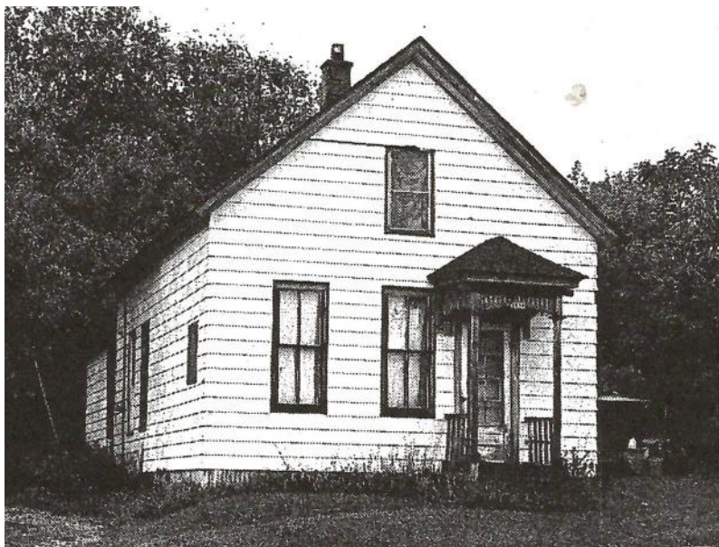
Above: Final photo of the Waiting Room before it burned by the fire department and was razed.
